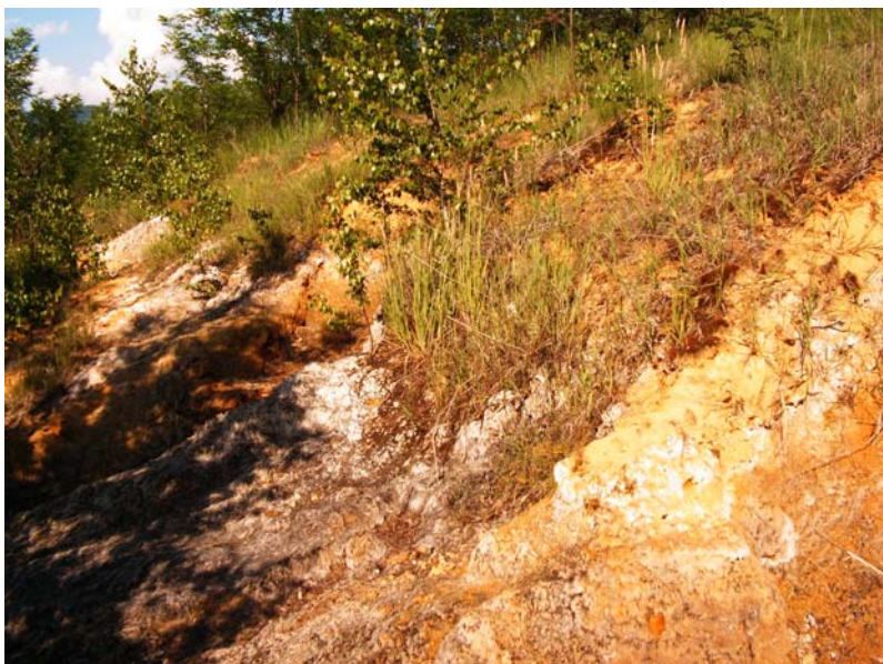
Figure 2. Ravines in the pond's dam
