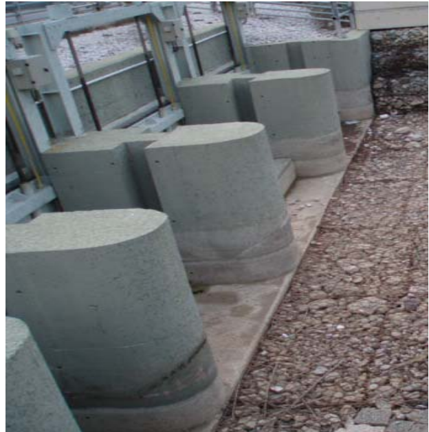
Fig. 4. Gate of the Channel connecting the two Lakes, Big Prespa and Small Prespa
